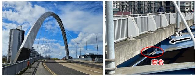
写真-8 Clyde Arc Bridge (全景と継手部の腐食)
