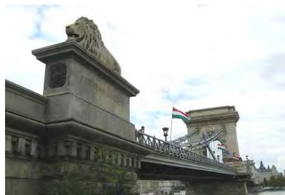
写真- 18 Széchenyi Chain Bridge
