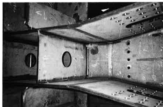
写真-7 溶接外観
